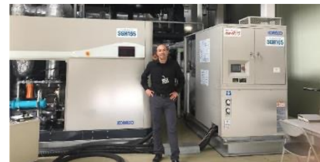
Kobelco SGH 120/165 (Steam Grow Heat Pump)
